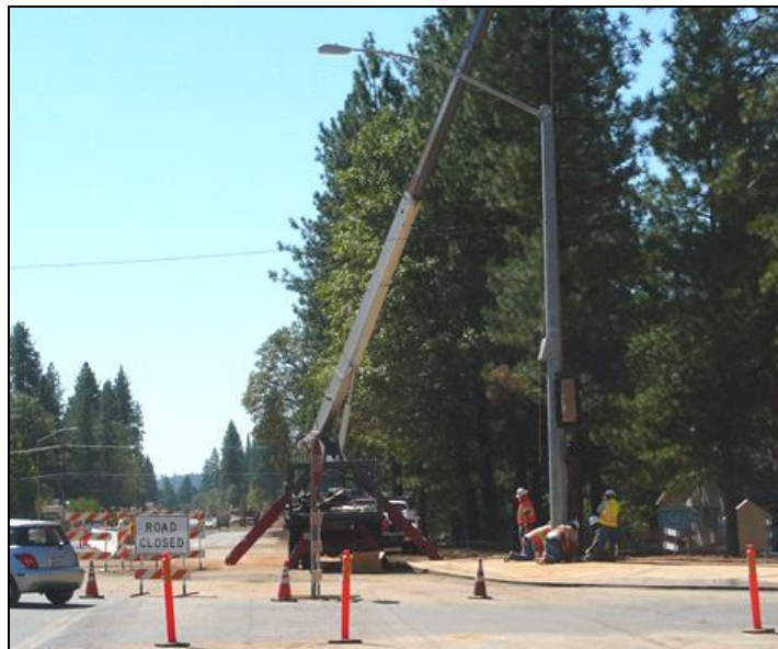
Light pole installed that will have traffic signal arm attached at SR 49 / frontage road intersection
