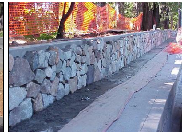
Stone retaining wall being constructed on Zion St.
